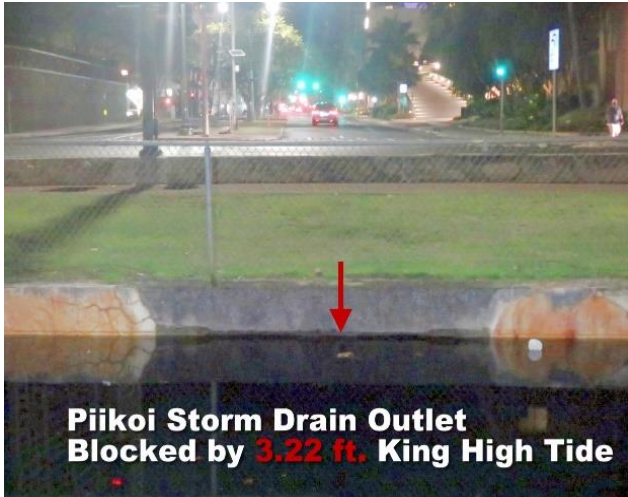
Photo 10 - 9:12 pm - 0.05-ft. Low tide Piikoi storm drain under Ala Moana Blvd. Photo 11 - 5:38 am 3.22-ft. King Tide. The 5:06 am 3.22-ft. King High Tide still covered the storm drain outlet after receding already for one-half hour.
