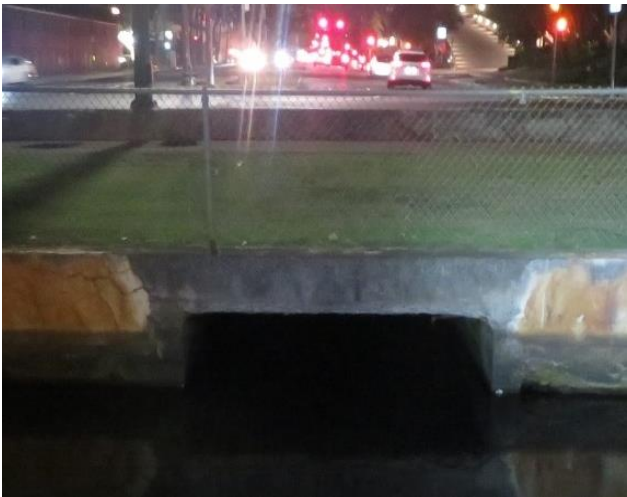
Photo 10 - 9:12 pm - 0.05-ft. Low tide Piikoi storm drain under Ala Moana Blvd. Photo 11 - 5:38 am 3.22-ft. King Tide. The 5:06 am 3.22-ft. King High Tide still covered the storm drain outlet after receding already for one-half hour.
