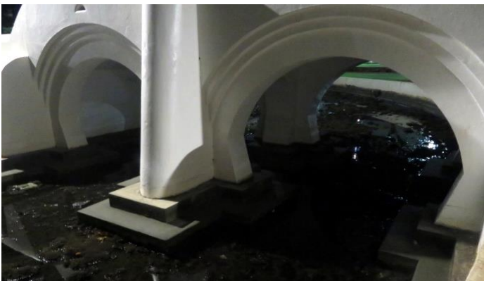
Photo 15 - 8:49 pm 0.05-ft. Low tide (water level 1") Kahanamoku pond bridge . Photo 16 - 5:57 am 3.22-ft. King Tide (water level 11" below top of banks). At 0" low tide, water would have basically drained from the canal if its bottom were cleaned.
