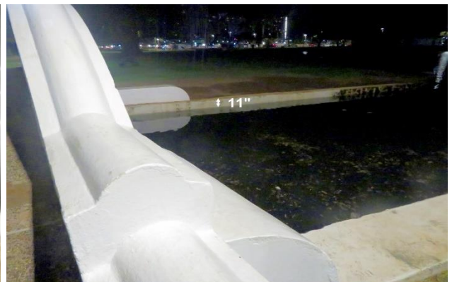
Photo 15 - 8:49 pm 0.05-ft. Low tide (water level 1") Kahanamoku pond bridge . Photo 16 - 5:57 am 3.22-ft. King Tide (water level 11" below top of banks). At 0" low tide, water would have basically drained from the canal if its bottom were cleaned.
