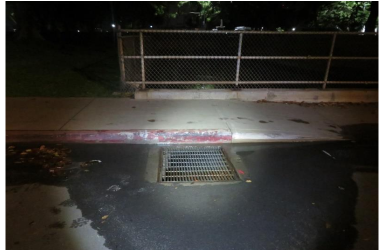
Photos 4, 5 – Dec.5, 2021, 4:43 am - Runoff from early morning lawn irrigation caused minor flooding along Ala Moana Park Drive as the 3.22-ft. King High Tide had risen from below to the base of the drain inlet.
