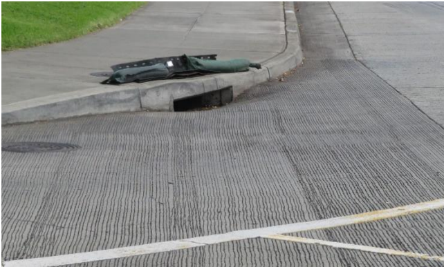
Photo 12 - Curbside storm drain street inlets... Photo 13 , if clogged, cause immediate flooding (Dec. 6, 2021 10:10 am).
