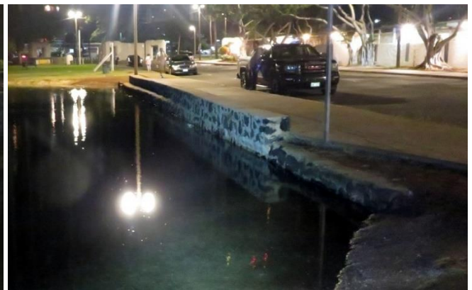
Kahanamoku canal inlet/outlet at Ala Moana Park Drive. Photo 21 – 5:17 am 3.22-ft. King Tide
