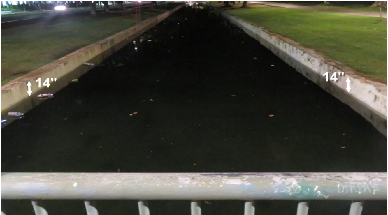
Photo 14 -5:35 am - Looking east from the Piikoi Park Bridge along 4-foot-deep and 26-foot-wide Ala Moana Blvd. canal. The 5:06 am 3.22 ft. King High Tide of Dec. 5 th , 2021 has risen to within 14" of the top of the banks.
