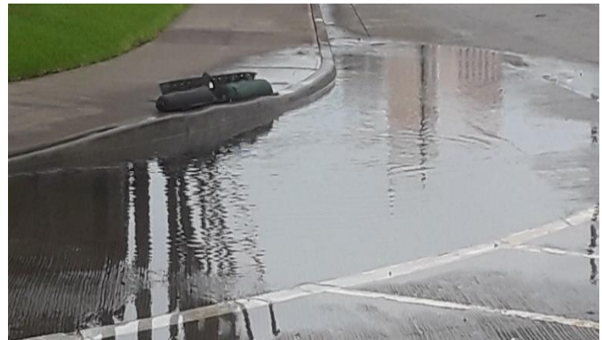
Photo 12 - Curbside storm drain street inlets... Photo 13 , if clogged, cause immediate flooding (Dec. 6, 2021 10:10 am).
