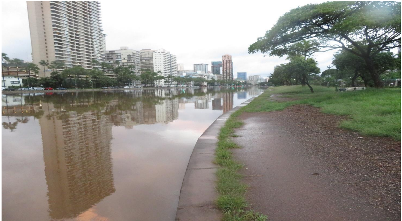
Photo 37 – 7:09 am – Flooded canal banks as the Manoa-Palolo Flood Control Canal discharges into Ala Wai Canal. Storm runoff from earlier rain showers in the mountain watersheds (prior to about 4:30 am) kept the water level elevated above the 5:42 am, 2.86-ft. King High Tide even 90 minutes later.
