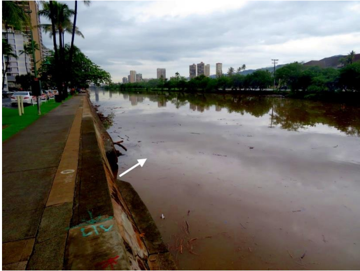
Photo 2 - 11:27 am. No rain yet. No pollution from storm drain. Photo 3 - 12:02 pm. Pollution plume- 24 minutes of rain. Paoakalani Ave. Storm drain outlet at 0.33-ft. low tide. Water level 19" to top of storm drain outlet, 65" to water level.
