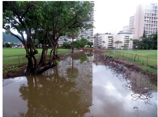
Photo 31 - 7:00 am...leading over drainage canal.
