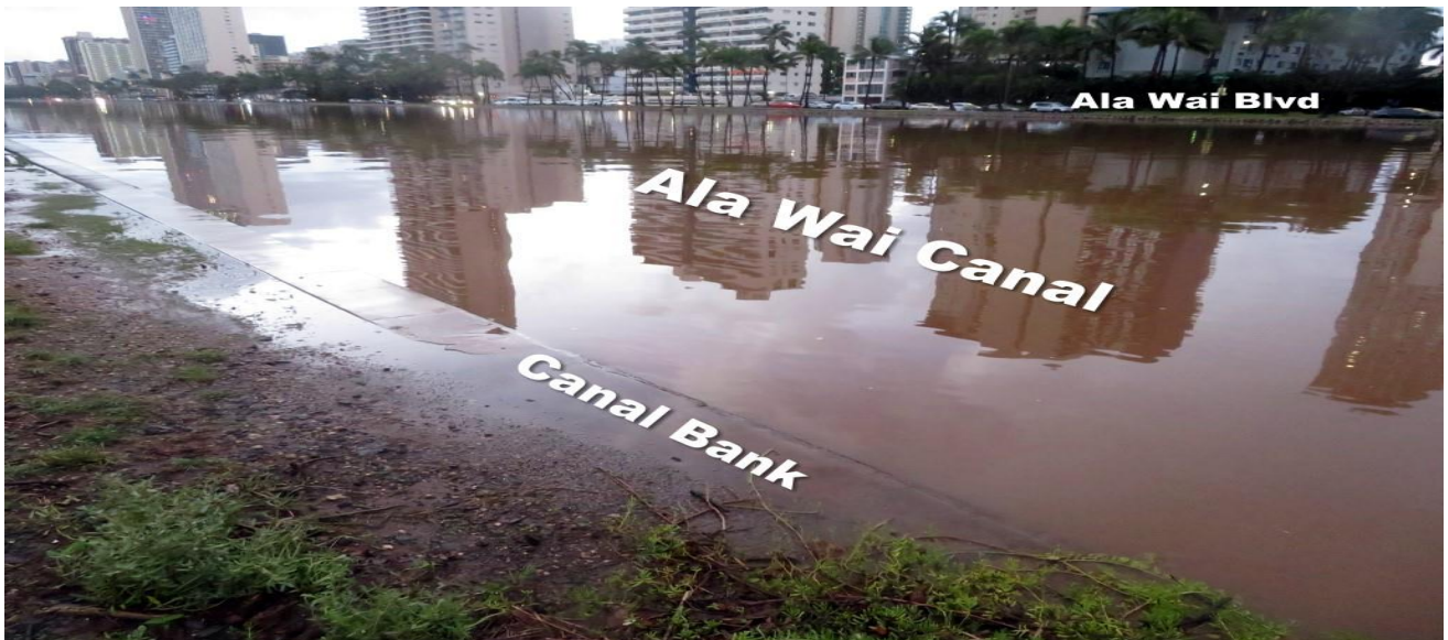
Photo 32 - 7:01 am – Flooded Ala Wai Canal banks along the Ala Wai Neighborhood Park.
