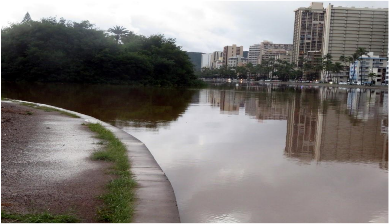
Photo 38 - 7:14 am – Manoa-Palolo Drainage Canal flooded side banks as it discharges into the Ala Wai Canal across from Lewers Ave. and just downstream of Seaside Ave.
