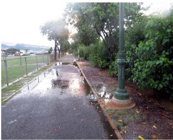
Photo 42 - 7:17 am - Flooded park walkway
