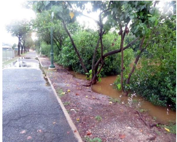
Photo 41 - 7:17 am - Flooded Manoa-Palolo Drainage Canal banks.
