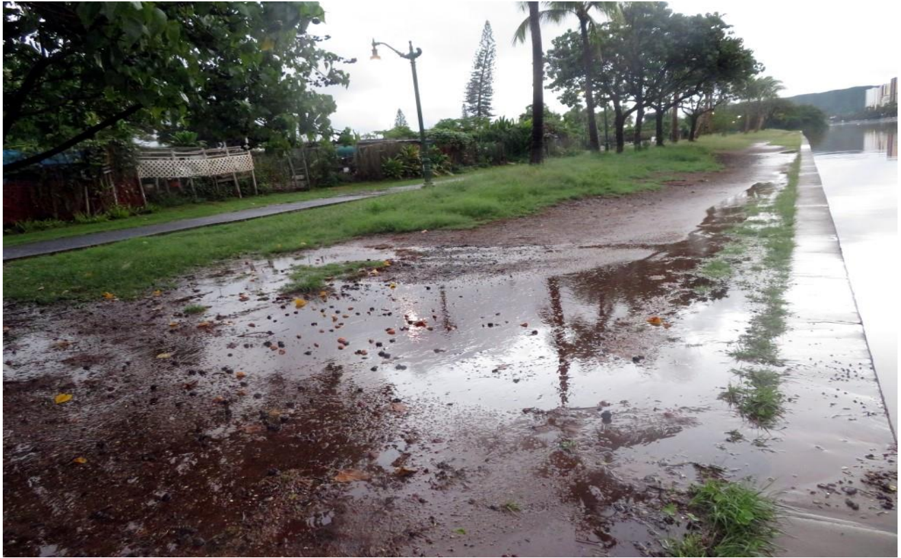
Photo 36 - 7:09 am - Flooded Ala Wai Canal side banks near the Ala Wai Community Garden.
